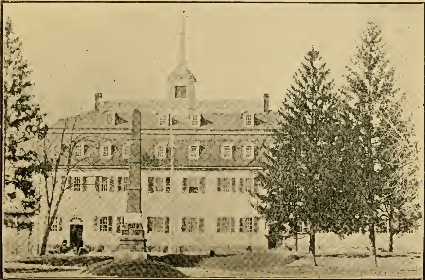
NAZARETH HALL, NAZARETH, PA. Moravian Boarding-School for Boys, Erected 1755
