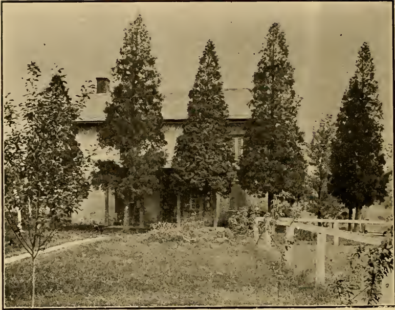
THE BLUMER HOUSE NEAR THE IRON BRIDGE
