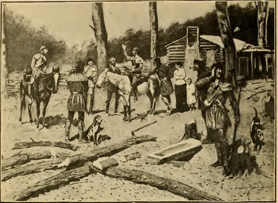
"COURIERS CARRIED THIS APPEAL THROUGHOUT THE COUNTRY"
