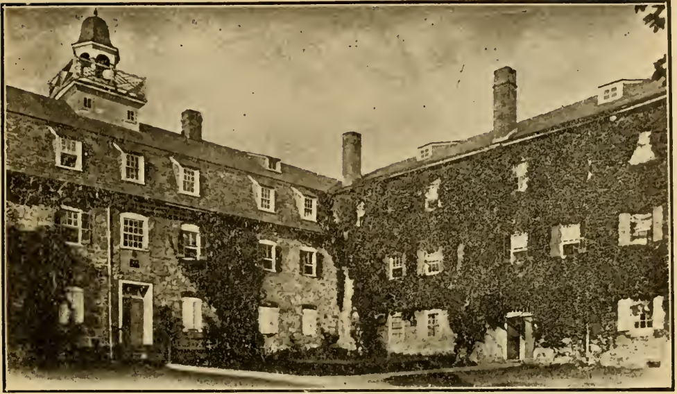
FIRST PERMANENT CHURCH-SCHOOL BUILDING AT BETHLEHEM, PA. Erected in 1749
