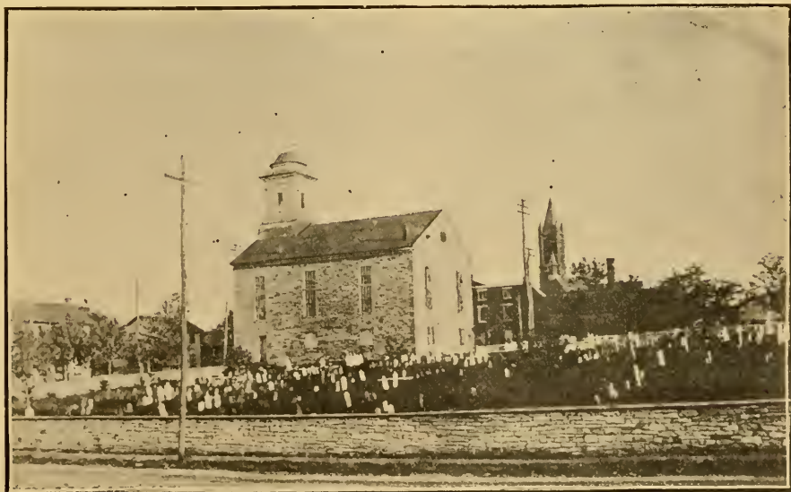
ZION EVANGELICAL LUTHERAN CHURCH, AT HUMMELSTOWN, PA. BUILT 1815-16
