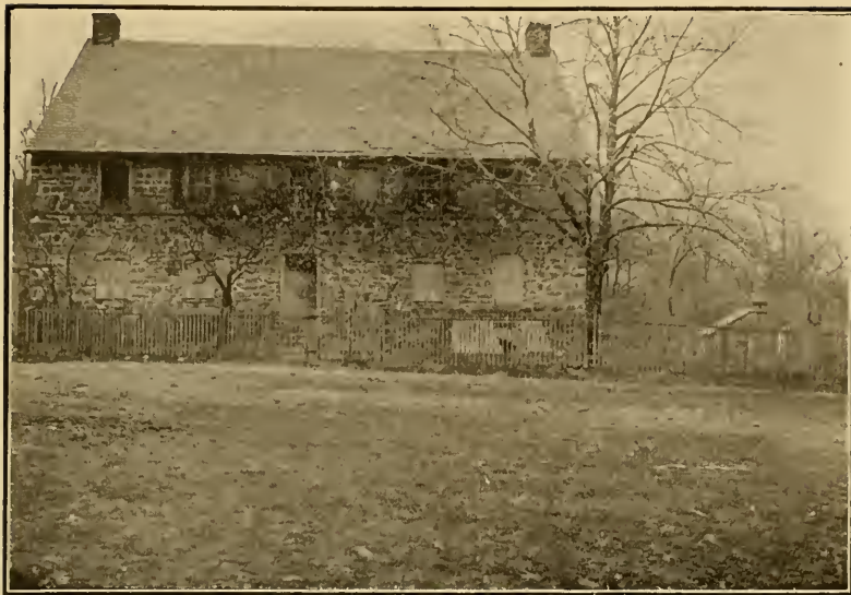
THE TRAXEL OR STECKEL HOUSE NEAR EGYPT, PA.
